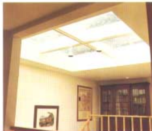
Unshaded skylights allow excessive heat and glare.
